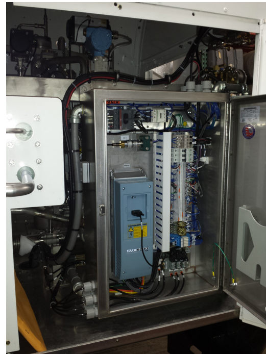
Heater is located behind VFD in electrical panel
